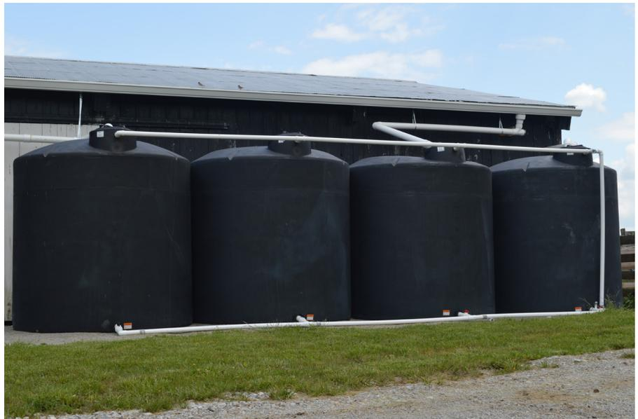
**Figure 3.** A series of aboveground tanks that have been connected together to create one large storage system. Valves on the pipes coming out of the bottom of each tank allow tanks to be drained and managed individually, if necessary. A common overflow pipe plumbs overflow water from the tanks outside of the production area. Similar concepts may be applied to cisterns. Photo by Lee Moser
